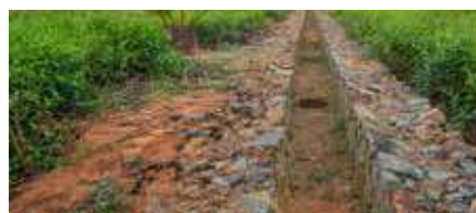
Drainage and sediment control system introduced at Millakande Estate enhancing environmental protection and soil conservation.
