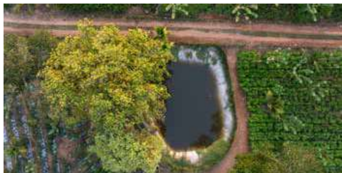
Millakanda Estate Rain Water Collection Pond
