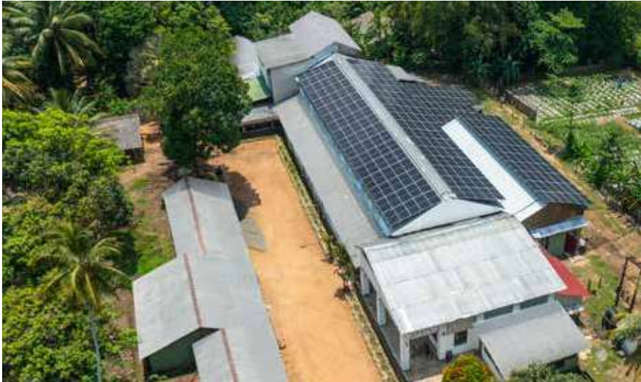
Factory rooftop solar installed at Frocester
