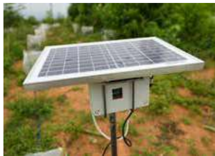
Smart weather station installed at Stockholm Estate.
