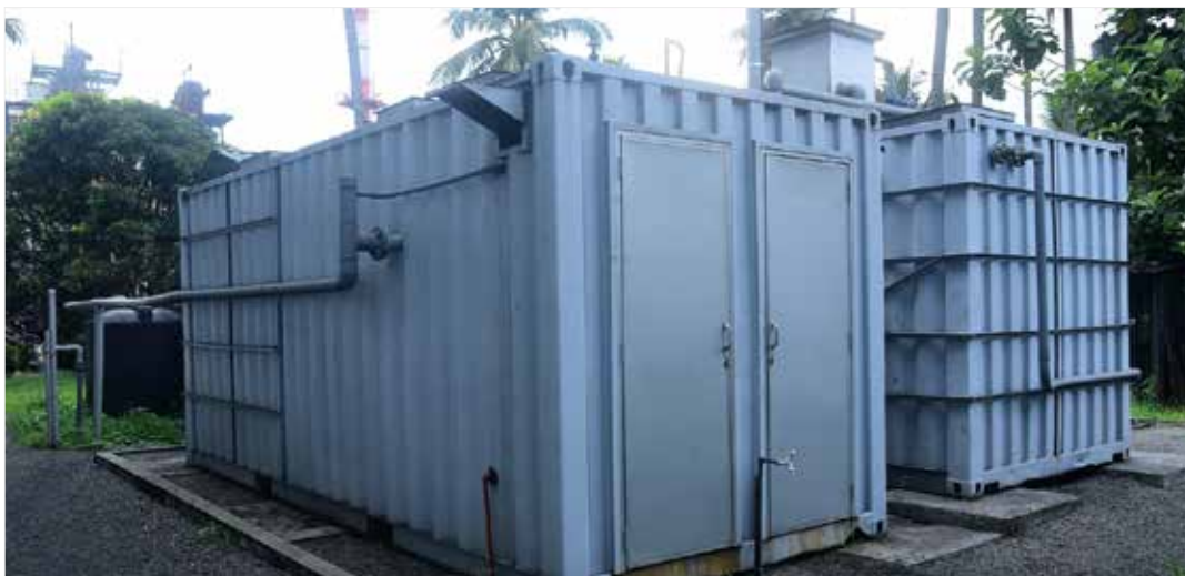
Containerized wastewater treatment system
